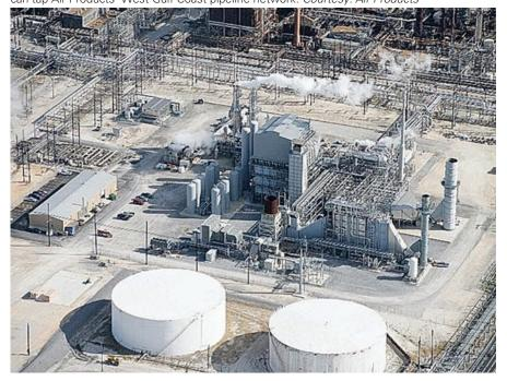
The refinery, on a 4,000-acre site about 90 miles east of Houston, needs all of those inputs because it's big and versatile. It converts more than 300,000 barrels a day of crude oil (including 100% sour crude) into jet fuel, low-sulfur diesel fuel, petrochemical feedstocks, petroleum coke, and conventional and reformulated gasoline.
