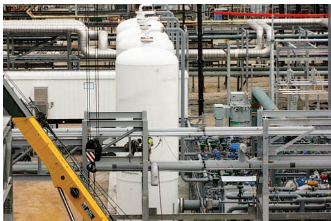
FIG. 4. VSA trains are used to remove more than 90% of the CO 2 contained in the reformer PSA feed gas.
